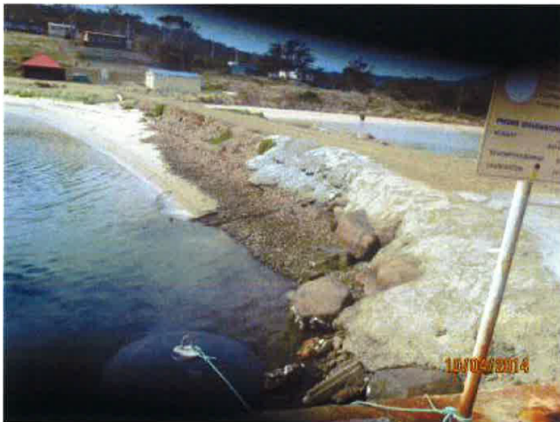
Figure 8.4.1 – Northern side of approach embankment requiring new rock armour
