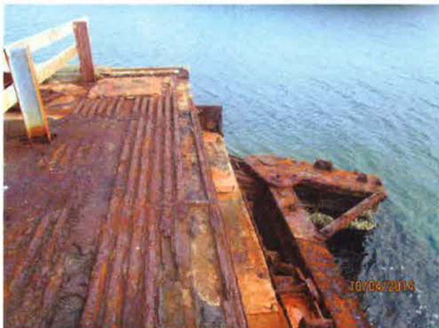
Figure 8.4. 5 – Exposed steel work at northern end
