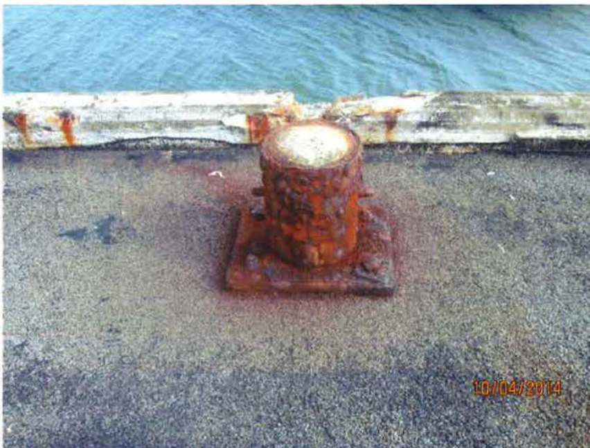
Figure 8.4. 7 – Corroded bollards
