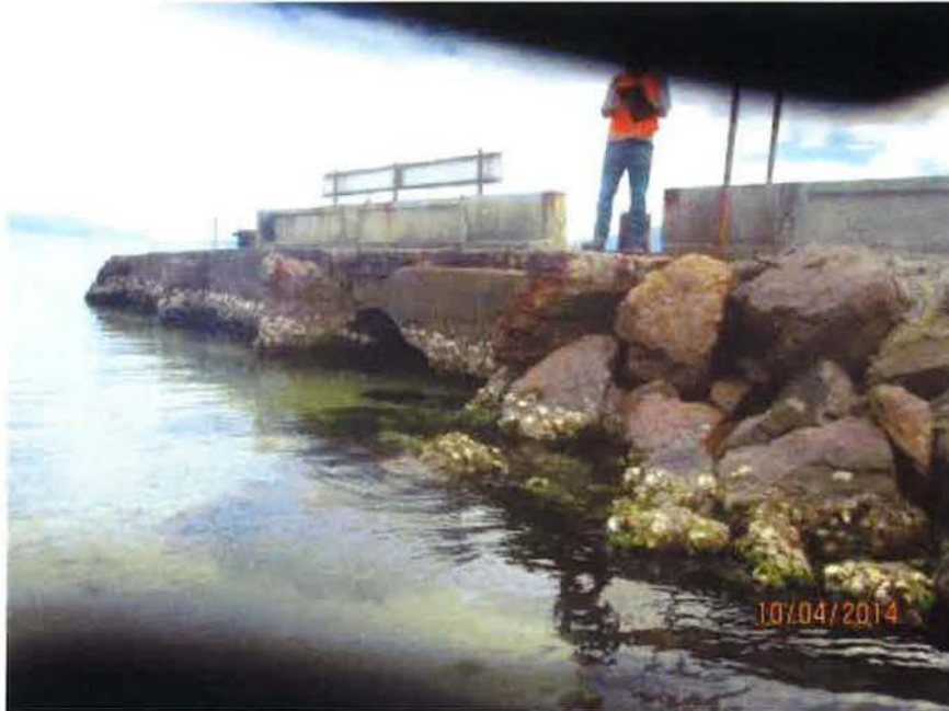
Figure 8.4.2 – Southern rock armour proposed for extension (accessible chamber in front of where person is standing).
