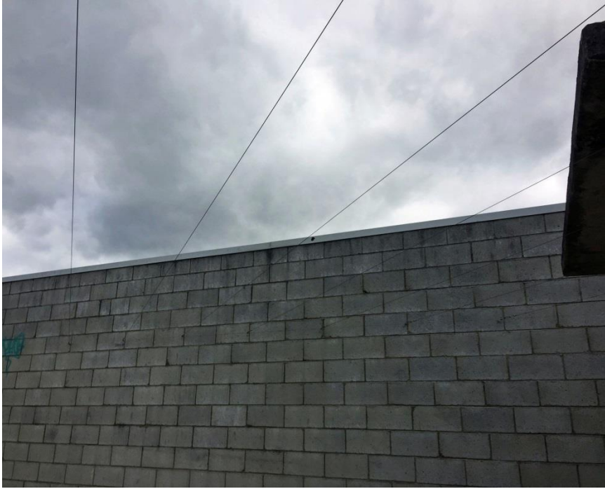
Detail of the stainless steel wires where the Artwork will be installed
