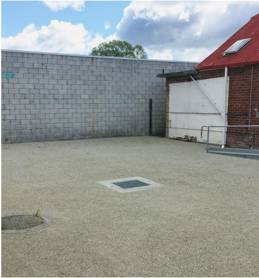
The corner of The Courtyard where the installation will occur
