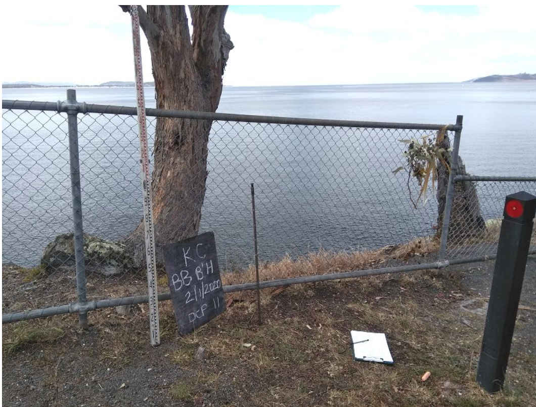
Figure 8. Different heights of the cyclone fence at the Talone Road carpark opposite the Blackmans Bay Blowhole (at DCP11). At left, the fence is 1.4m high; at right, about 0.9m. Abseilers anchor from this location. Anecdotal, an old couch was positioned at one time over the fence at left.
