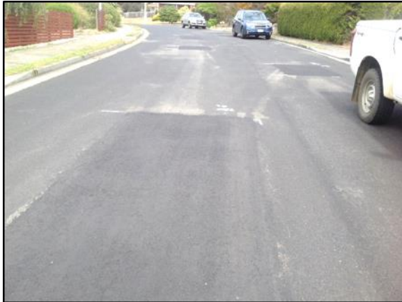
Crystal Downs Drive – reseal preparation
