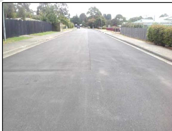
Endeavour Avenue – asphalt overlay
