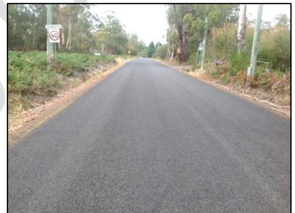
Howden Road – two coat seal
