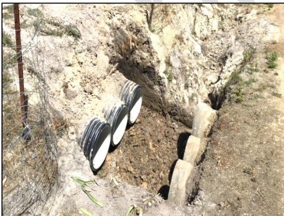
56 Tabors Road – stormwater culvert upgrade
