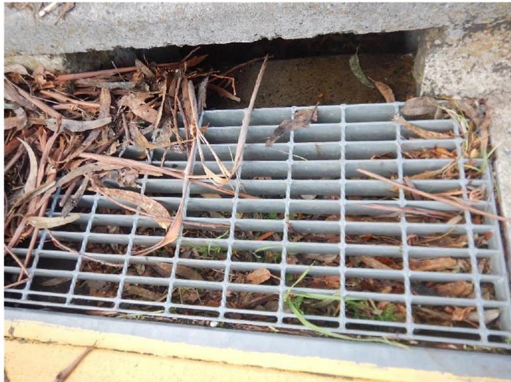
Figure 4.2 Example of Potentially Insufficient Pit Depth
