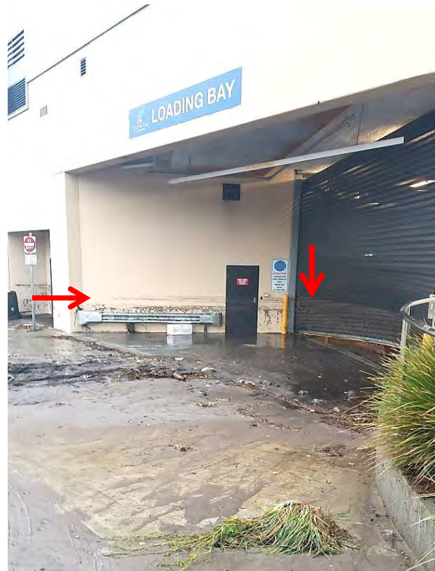
Photo 4: Debris Mark Measured at 1.17 m above Ground ( RL 27.5 m from DA Plans 2010) opposite 16 Freeman Street, Kingston
