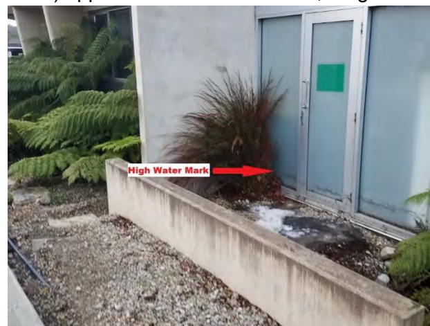
Photo 6: High Water Mark in Emergency Exit Door 0.25 m above Floor Level (Ground Floor Level = RL 15.0m in 1996 Original Drawings) at 15 Channel Highway, Kingston (Kingborough Civic Centre)
