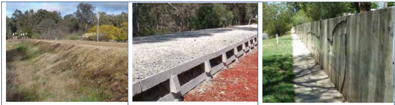
Photo 24: Earthen Embankments (L), Crib Walls (M), and Concrete Retaining Walls (R)
