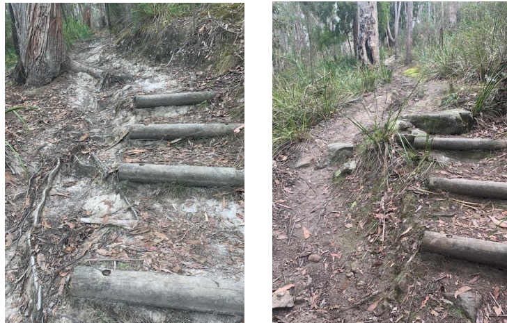
Example of erosion on a section of Nierinna Creek Track steps
