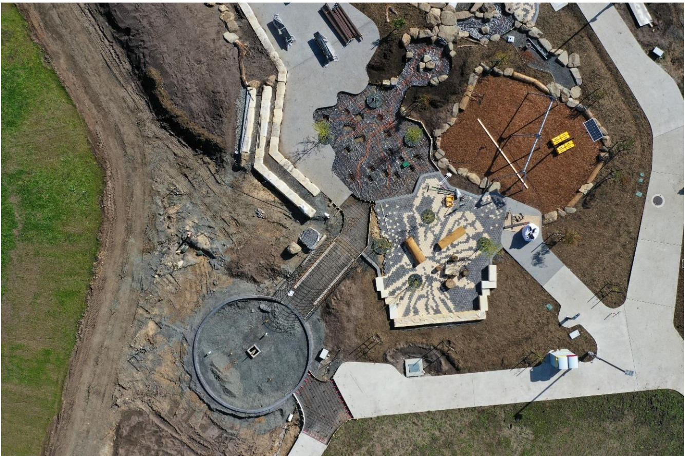
Figures 14a & 14b – Construction as at October 2020
