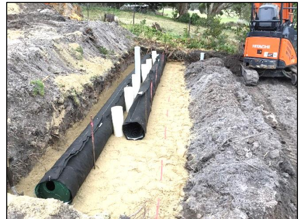
Alonnah – septic waste absorption bed upgraded
