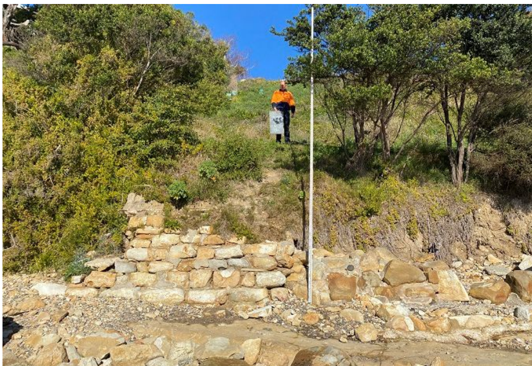
Figure 2. The mortared sandstone seawall originally protected almost the full 170m of track described in this report. It contains sandstone blocks ranging in length from about 0.2 – 0.6m, and about 0.25m wide and high (approx. 20 – 100kg). Wave action has destroyed almost of it. The staff is 5m high.
