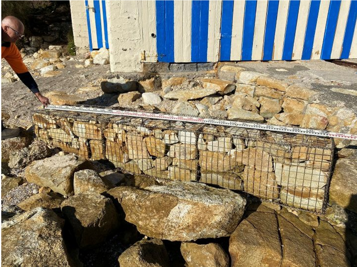
Figure 7. A 3m long gabion of on-site sandstone blocks encased in a high-strength stainless steel cage has survived intact on the rock platform at the boatshed near chainage 170m. Similar gabions are suggested as an aesthetically acceptable coastal defence from chainage 0 – 170m to mitigate embankment erosion.
