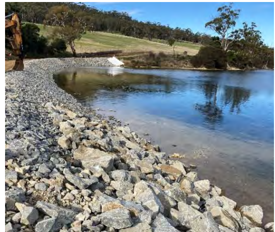
New revetment under construction
