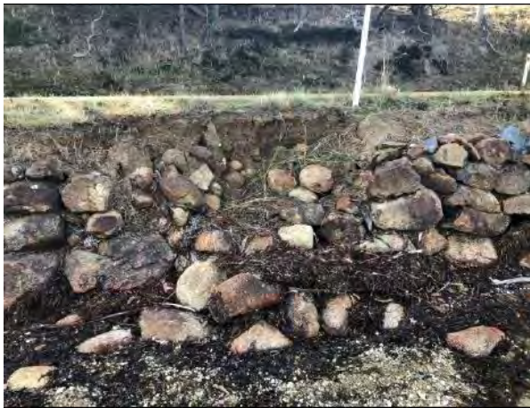
The failing rock wall
