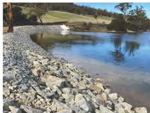
New revetment, Missionary Road, Barnes Bay
