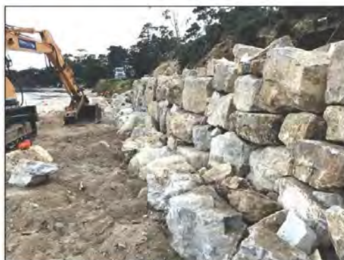
Repairs to retaining wall, Nebraska Road
