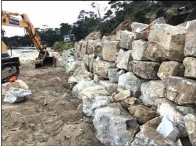
Repairs to retaining wall, Nebraska Road
