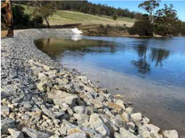
New revetment, Missionary Road, Barnes Bay
