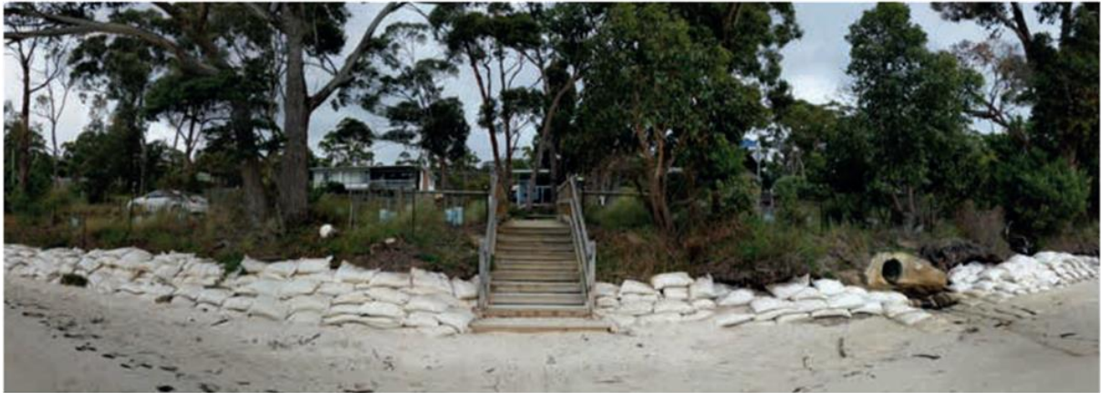
Sandbags now protect 65 metres of coastline at Coningham Beach in Kingborough Council.
