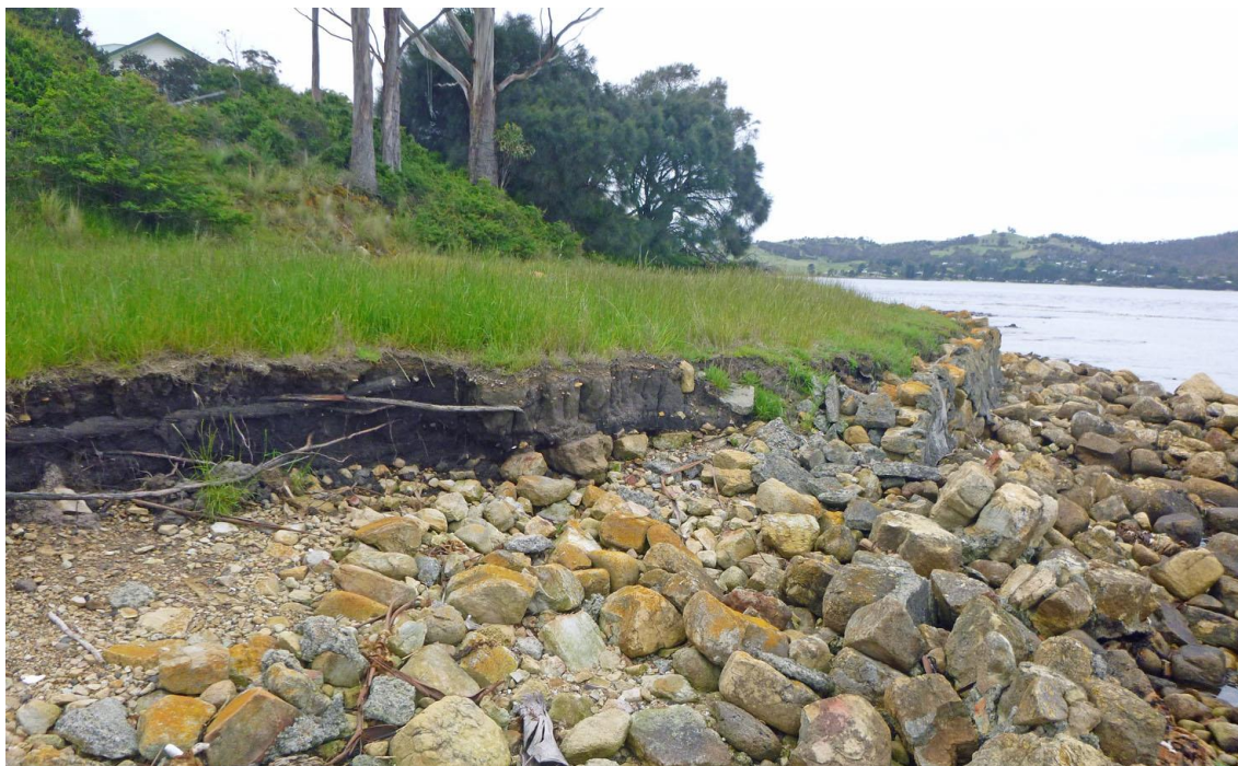
Figure 9: Artificial terrace on private land approximately 100 m east of Tinderbox Beach and jetty. Cement-and-stone seawall is intact on the right but has been destroyed by wave attack in the foreground – left. Recent wave erosion of the artificial terrace infill (soil) is apparent, with exposure of the roots of large living trees. Photo by C. Sharples 23 rd November 2021.
