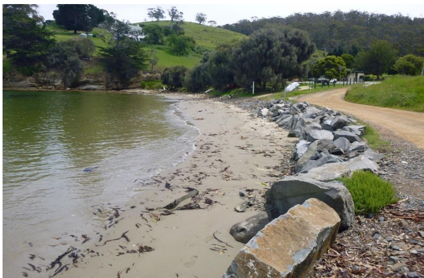
Figure 13: View west along Tinderbox Beach from the east end adjacent the Jetty. The dolerite boulder wall (‘revetment’) in the foreground protects the jetty access road, beyond which the eroding soil margin directly backs the sandy beach. Photo by C. Sharples 23 rd Nov 2021.
