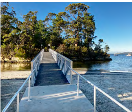
Popular Snug River footbridge replaced with a wider, longer-life aluminium bridge allowing for improved pedestrian movement and access.
