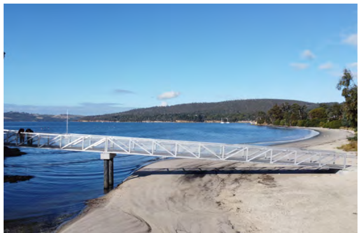
Popular Snug River footbridge replaced with a wider, longer-life aluminium bridge allowing for improved pedestrian movement and access.
