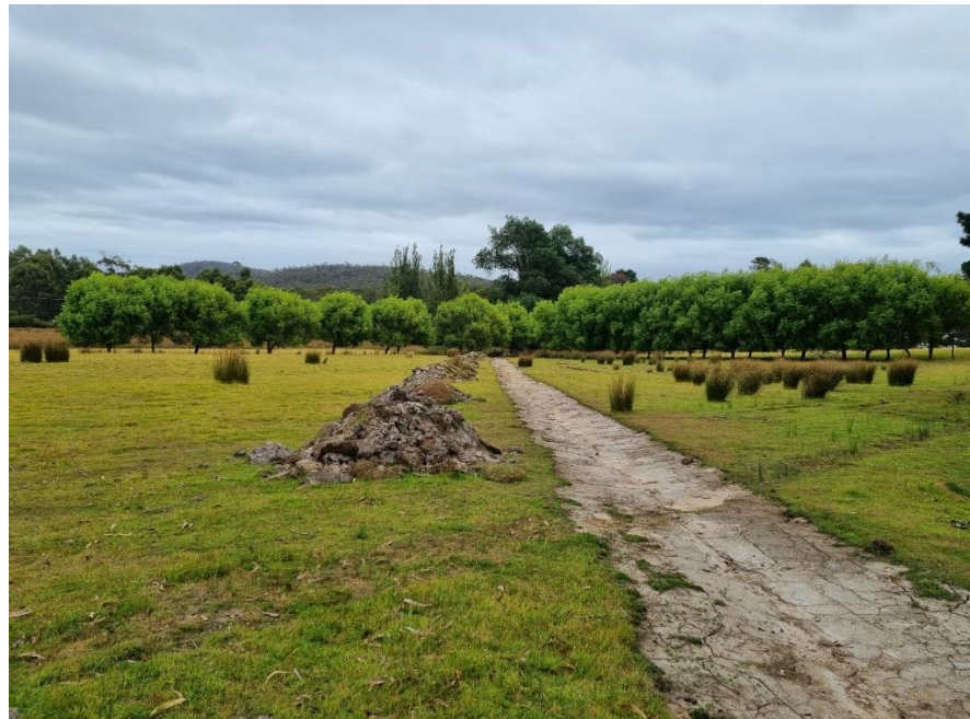
Figure 10: overflow trench from a neighbouring dam running through or close to the proposed building area on Lot 1
