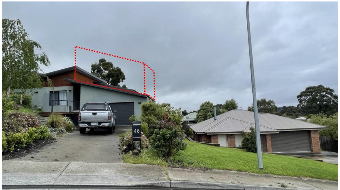
Figure 2 View of site from Jacaranda Drive (Source: site visit). NOTE: the proposed extension will sit above the existing garage – marked in red
