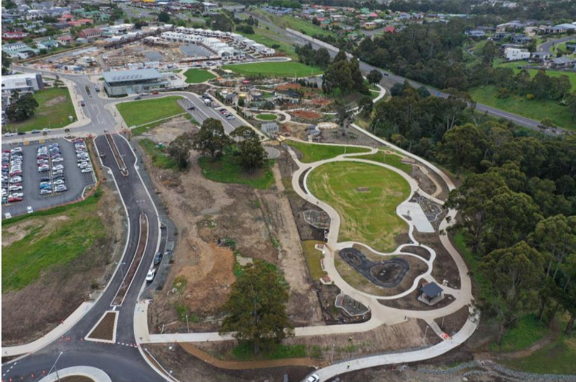
Figures 12a & 12b – site progress on P.O.S stage 2 - October 2022
