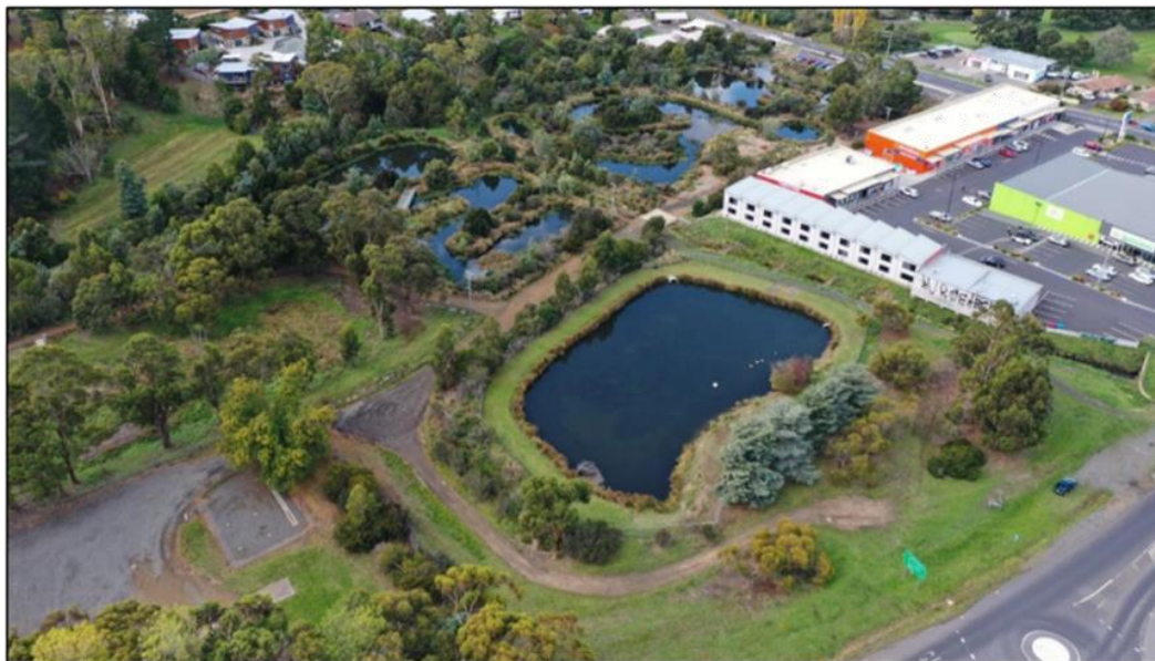
Figure 6 – Kingston Wetlands where upgrade works commenced in February 2023
