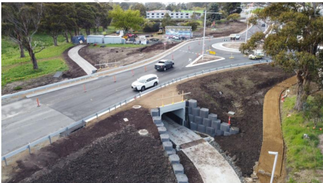
Figure 5 – New Huon Highway Pedestrian Underpass progress photo- October 2022.
