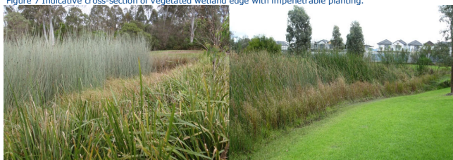
Figure 7 Indicative cross-section of vegetated wetland edge with impenetrable planting.
