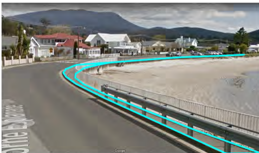
Photo 7: Proposed Sea Wall Upgrade – Raising the Footpath on Existing Sea Wall.
