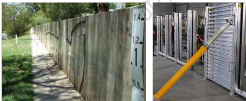
Photo 2: Concrete Retaining Walls (L) and Sliding Flood Gates (R).
