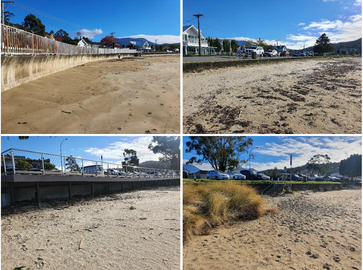
Photo 6: Existing Sea Wall along Kingston Beach.
