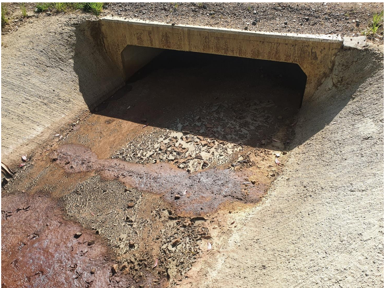
Figure 3. Box Culvert, Bundalla Road (site visit)
