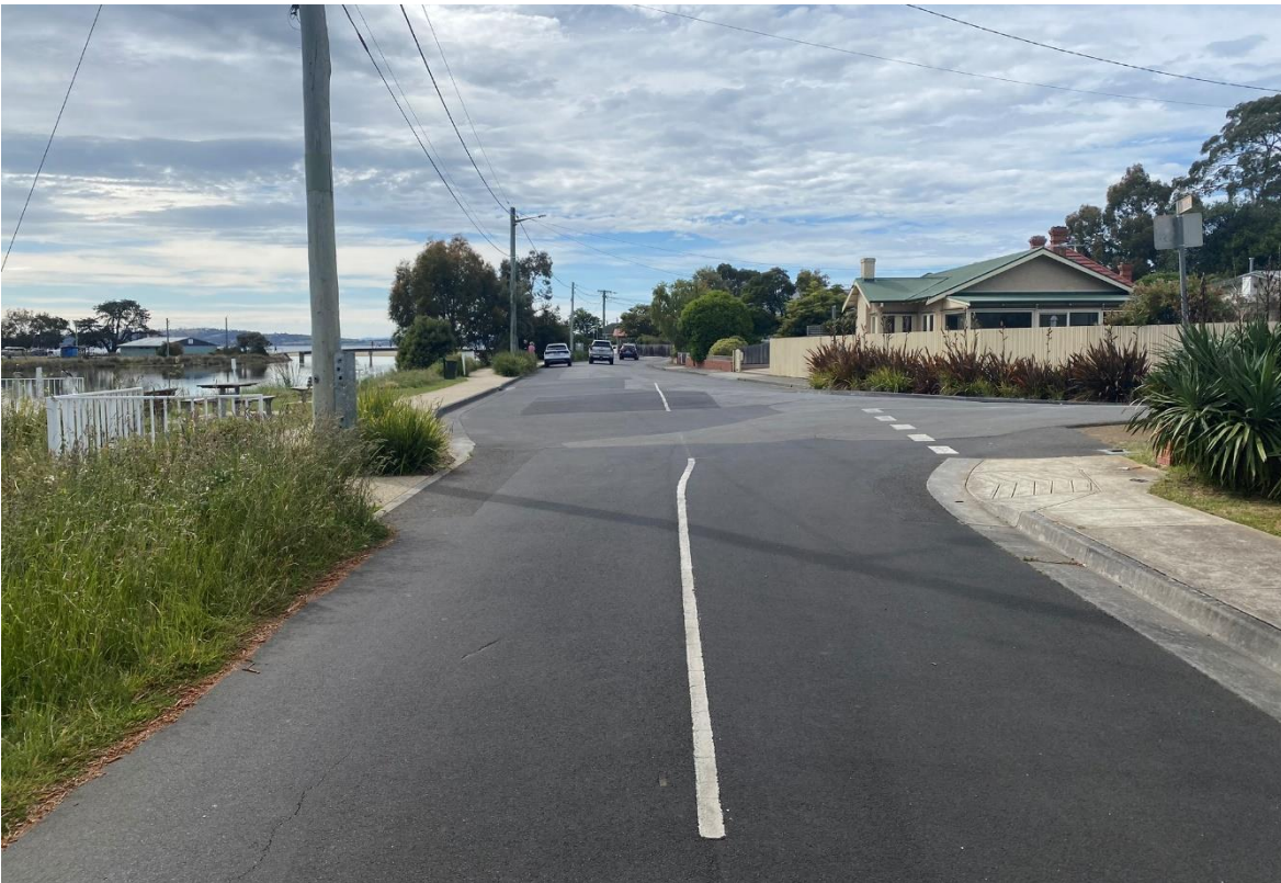
Figure B-18: Balmoral Road bend – view south-east towards intersection
