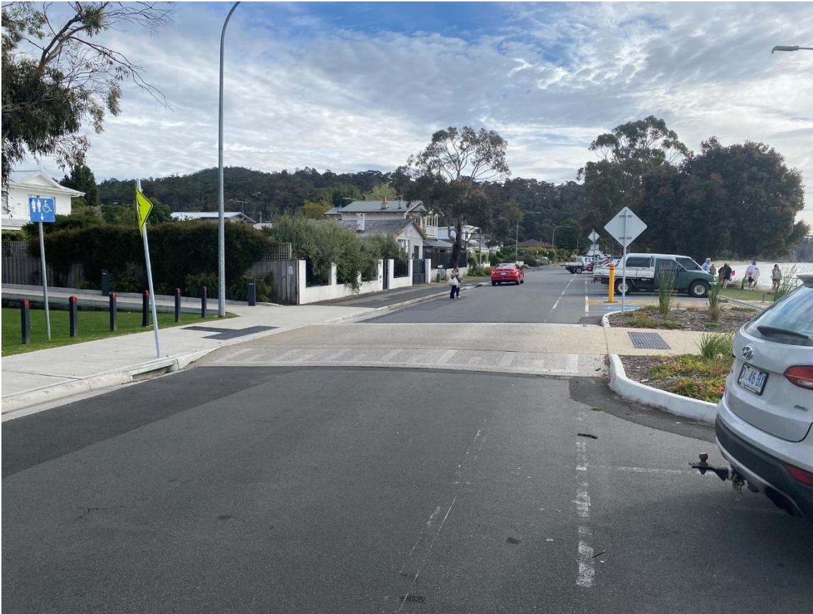
Figure B-7: Osborne Esplanade at Surf Life Saving Club – view north to crossing point
