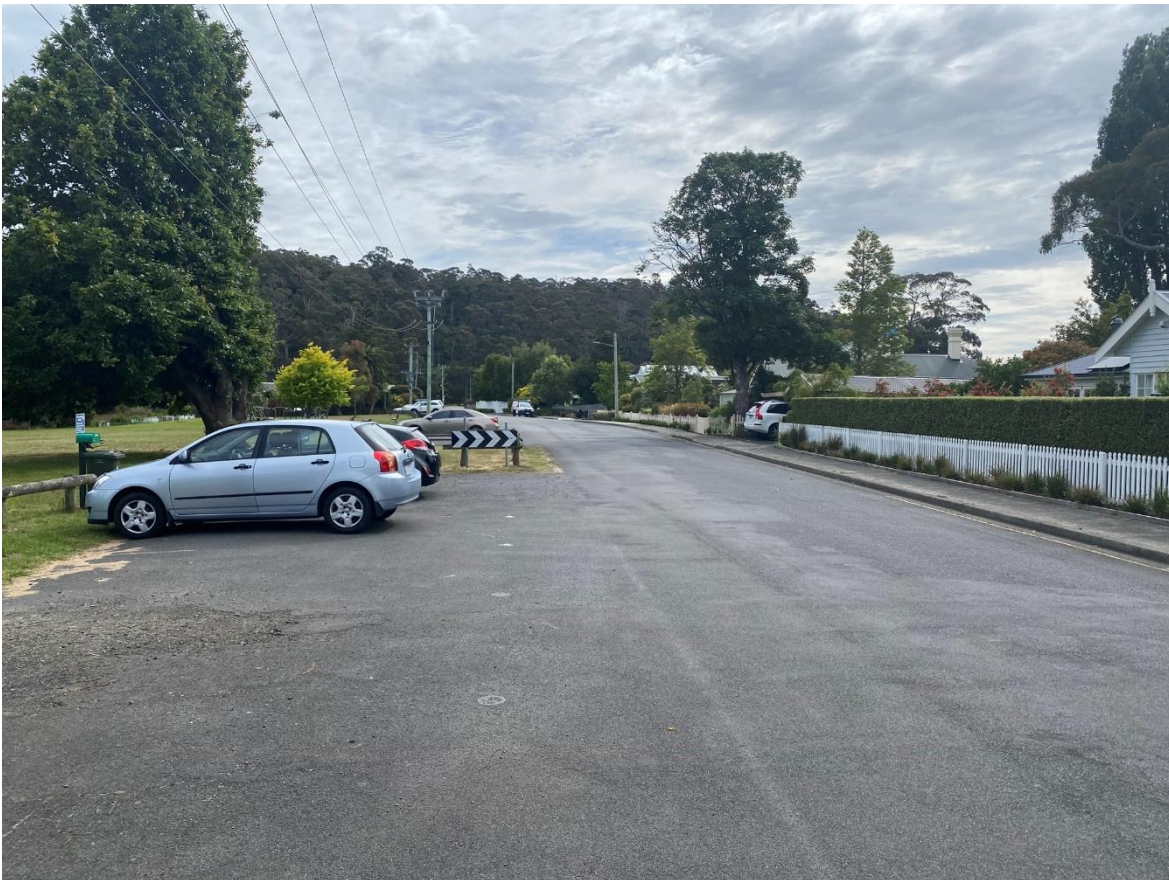
Figure B-16: Balmoral Road at Rotary Centennial Park – view north-east at informal parking
