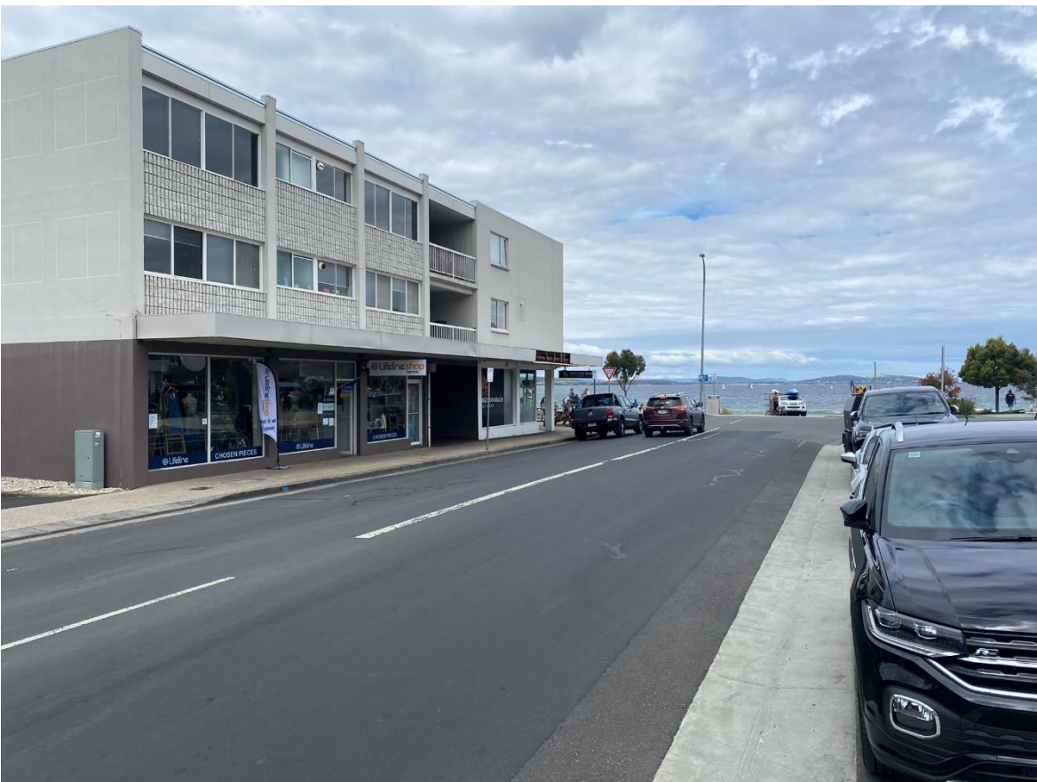
Figure B-6: Beach Road approach to Osborne Esplanade – view southeast
