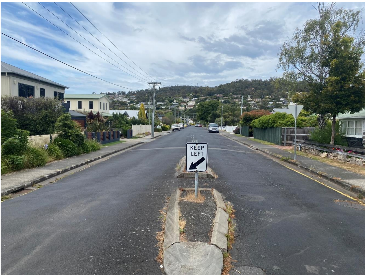
Figure B-22: Windsor Street at Victoria Street – view south-west
