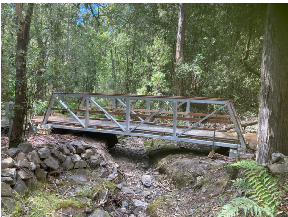
New Bridge on Nierinna Creek Track
