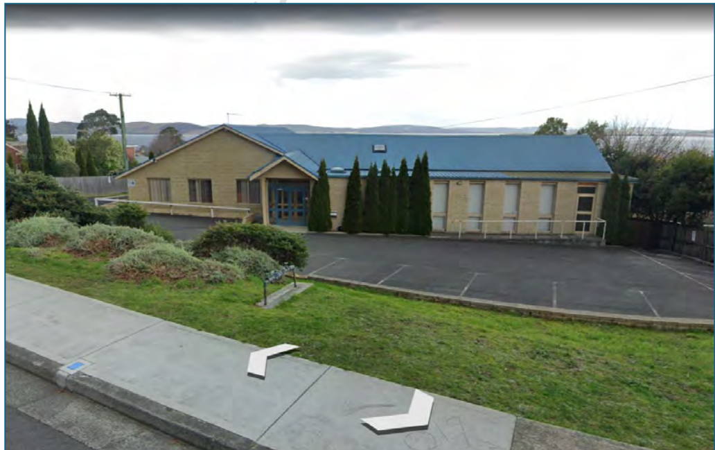
Figure 5 - Street view of 124 Chanel Highway (Ref: Google Earth).
