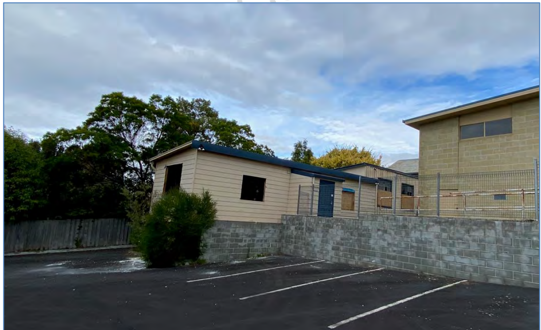
Figure 3 - Proposed buildings at rear of site to be demolished.
