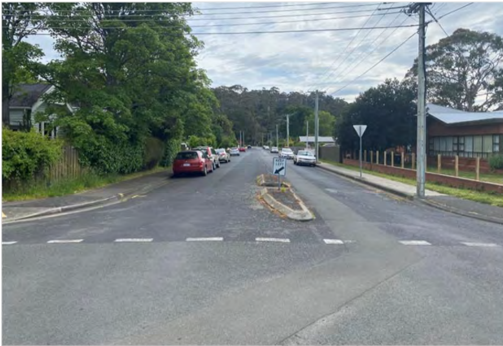
Figure B-21: Windsor Street at Victoria Street – view north-east
