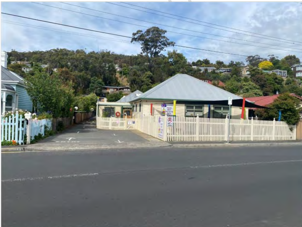
Figure B-24: View towards Kingston Beach Early Learning Centre Access off Beach Road
