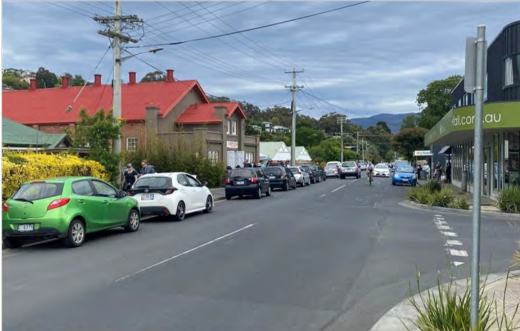
Figure B-2: Beach Road at Windsor Street – view west towards Kingston Beach Market activity
