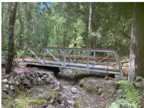
New Bridge on Nierinna Creek Track
