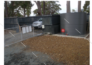
FIG 1: COMPLIANT STATIC WATER STORAGE & PROPERTY ACCESS
