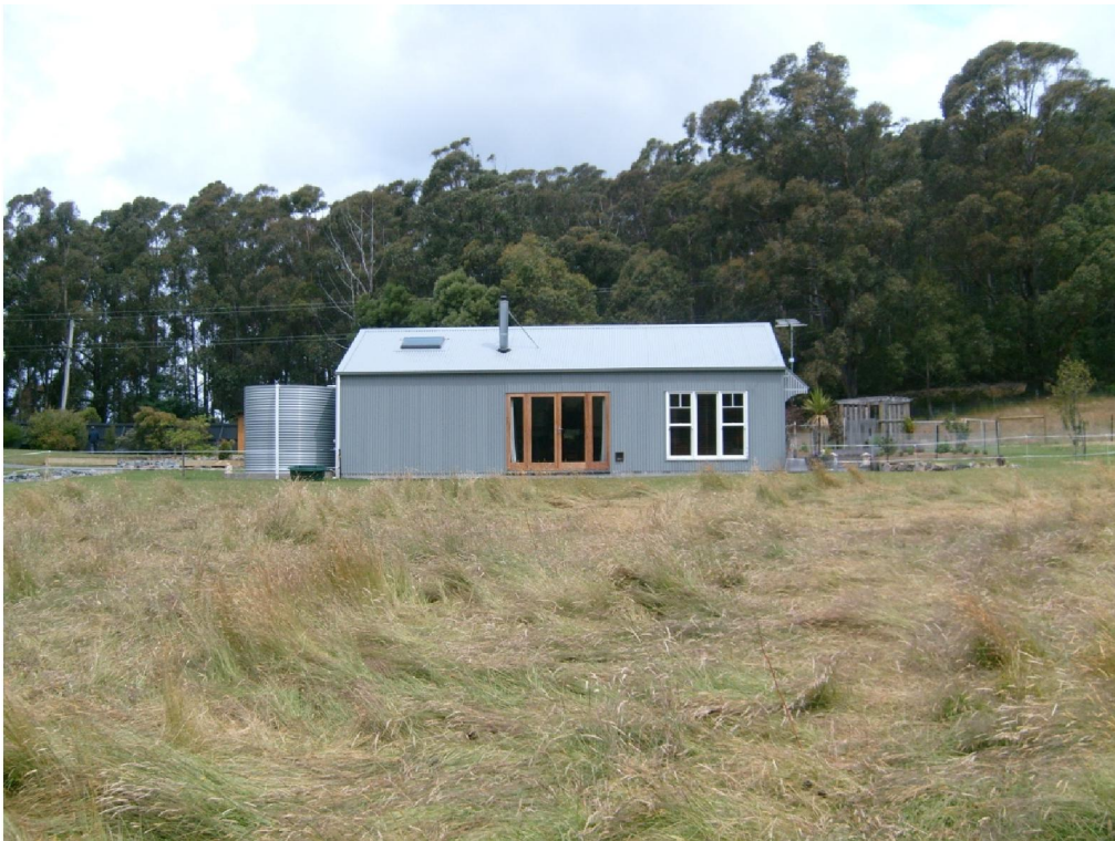
FIGURE 3: Looking south towards development site.
