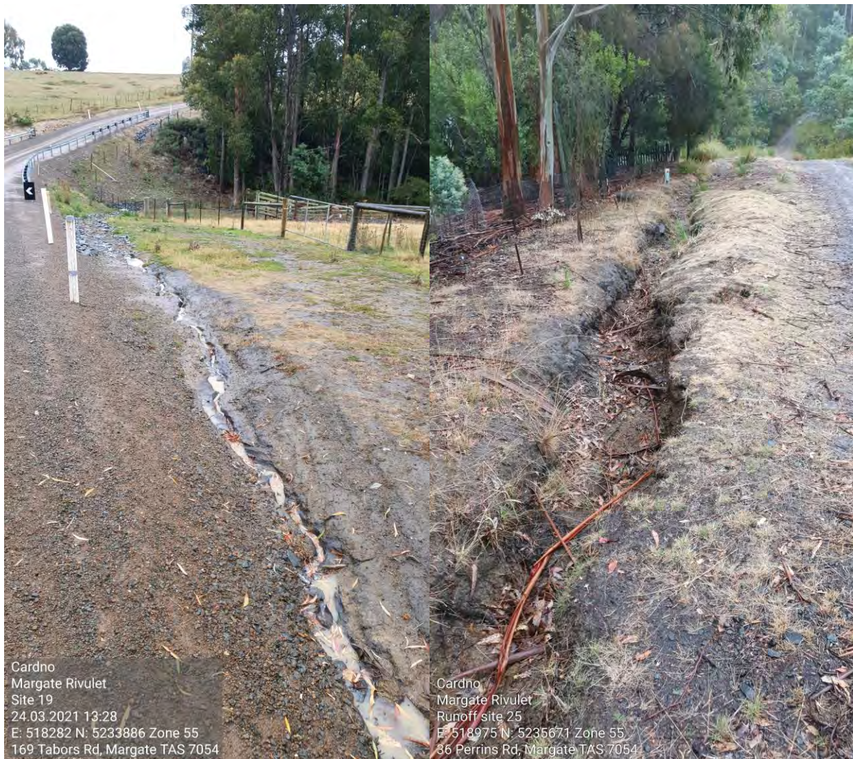
Figure 9-1 Examples of Erosion Observed During the Site Visit
