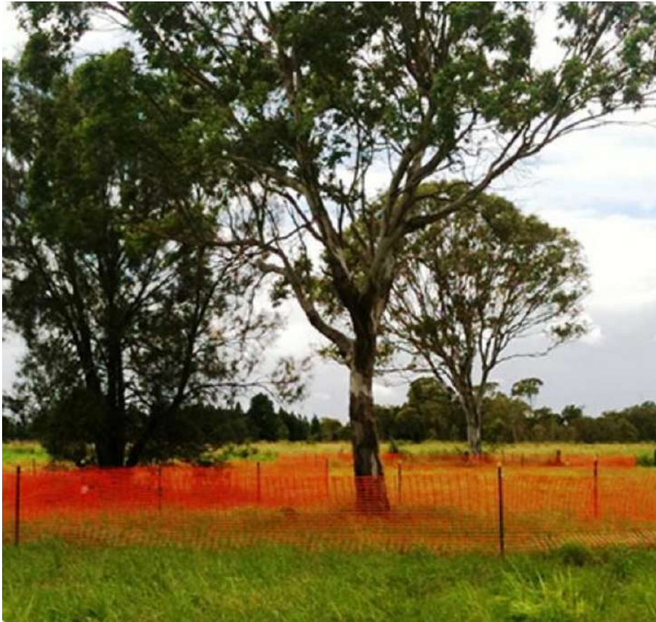
Figure 8- Tree Protection Fencing constructed with barrier mesh.
