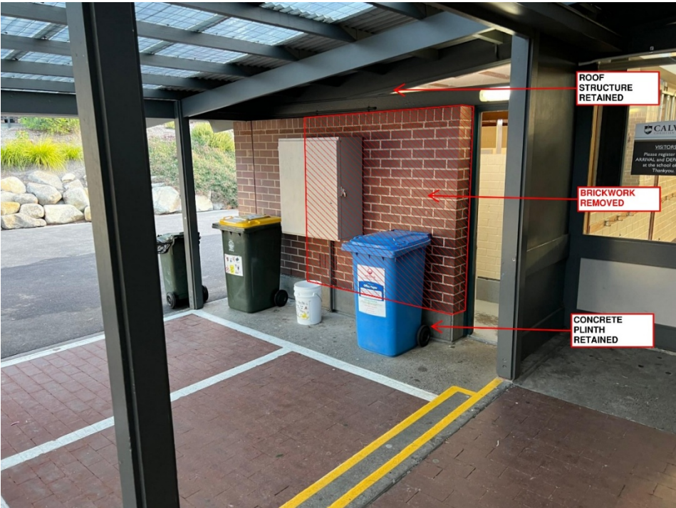
Figure 1. Existing photo with markups of proposed external works. Partial demolition of brickwork. Roof and plinth retained.
