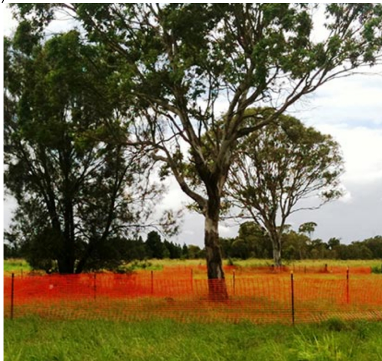
Figure 4- Tree Protection Fencing constructed with barrier mesh.
