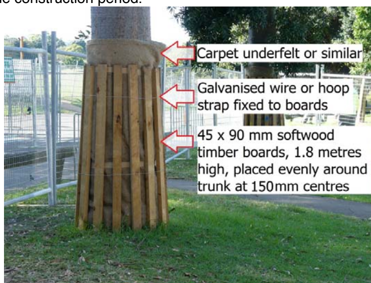
Figure 5- Example of tree trunk protection
